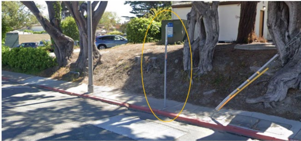
Bus Stop #6781 Cass/ Hartnell (City of Monterey) Category 2 – Sidewalk exists, but lacks passenger landing pad and clear path of travel
