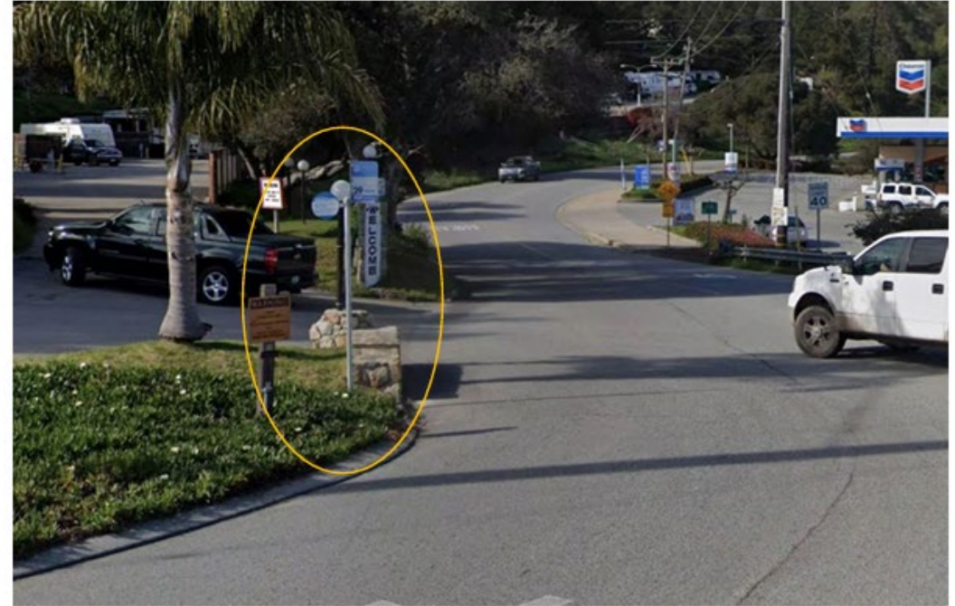
Bus Stop #2989 Prunedale North/ Highway 156 (County of Monterey) Category 3 – Lacks sidewalk and passenger landing pad
